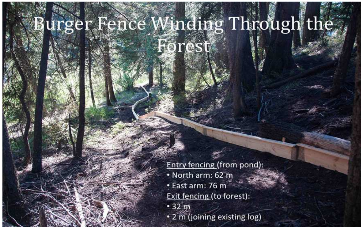
Figure 1. Drift fencing used in 2014 to funnel toadlets from the breeding pond uphill and through the underpass safely across parks road into the forest on the other side.
