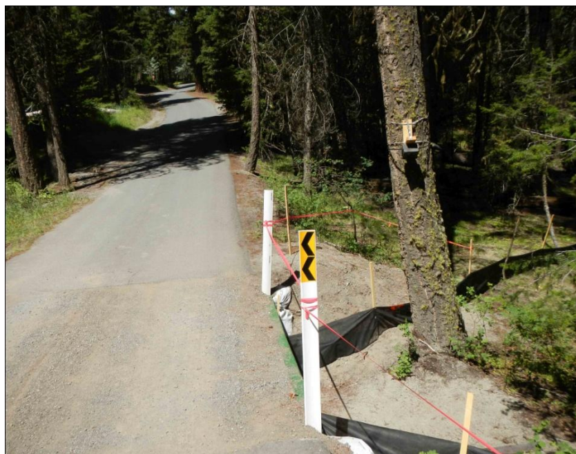
Figure 3. Overview of the underpass location and tunnel entry with drift fencing. Note the camera in the tree above the entry. The flagging was intended to keep curious by-standers at a distance.
